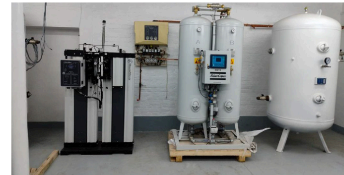
The newly installed oxygen plant
