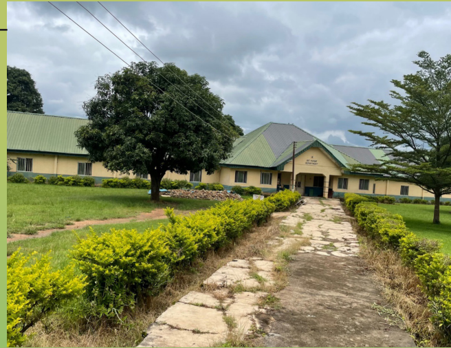
Jengre's School of Nursing during renovations
