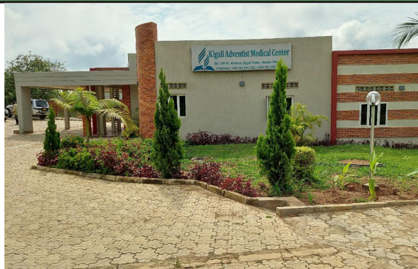
KAMC's newly renovated entrance and parking lot
