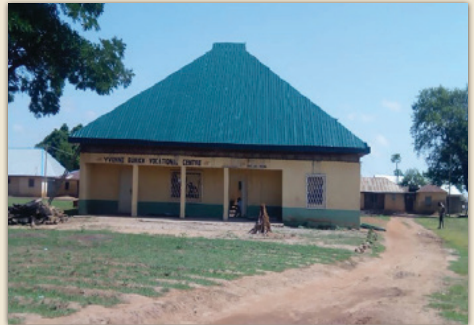
The Yvonne Eurick Vocational Center, located on the campus of Jengre Hospital in Nigeria, was recently renovated.
