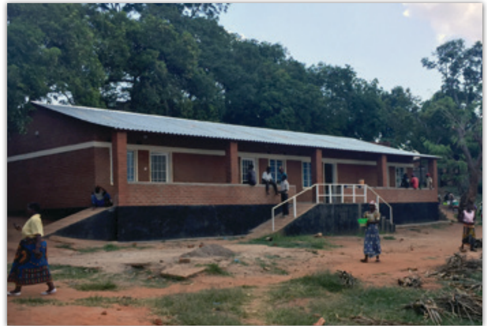
The recently completed Guardian Shelter at Malamulo provides living and cooking space for patient families.
