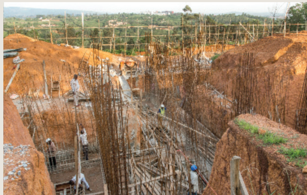
Construction has already begun on many of the AUCA support structures.
