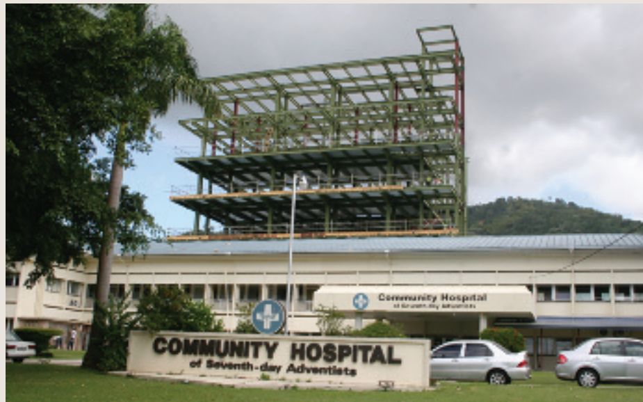
New construction at Community Hospital in Trinidad.
