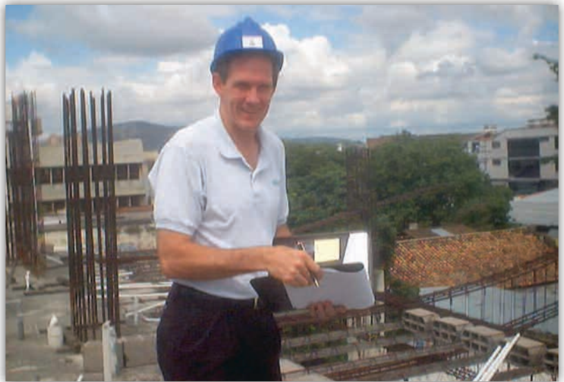
Ken Breyer inspects the new construction effort at Barquisimeto
