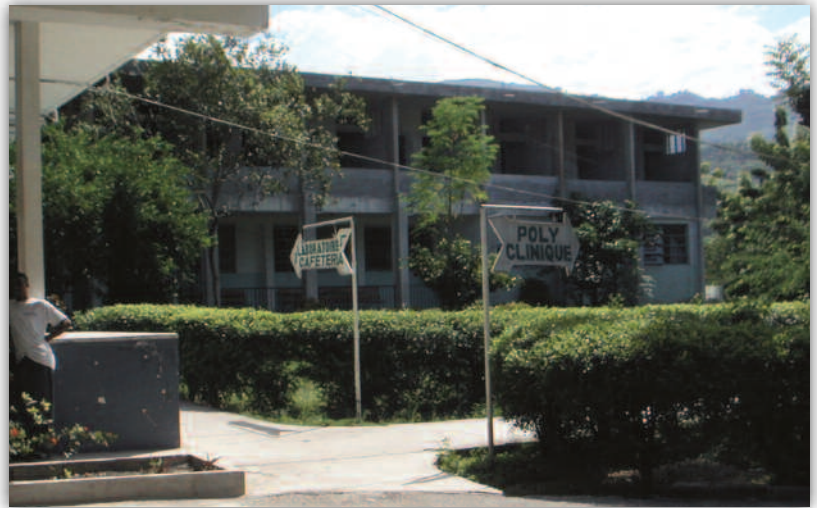
The new second floor wing nearing completion
