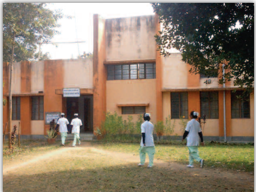
Nursing School Hostel in Ranchi
