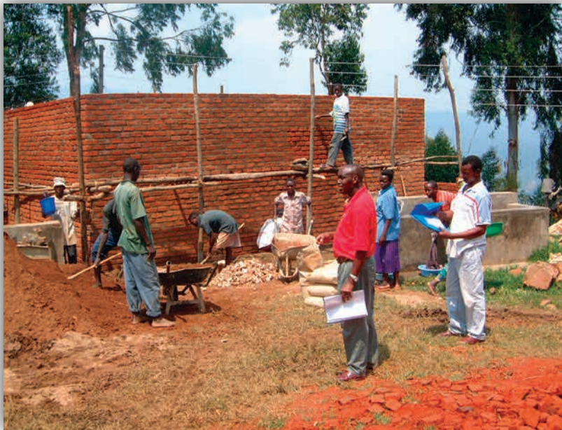
Patient cooking area nearing completion at Mugonero
