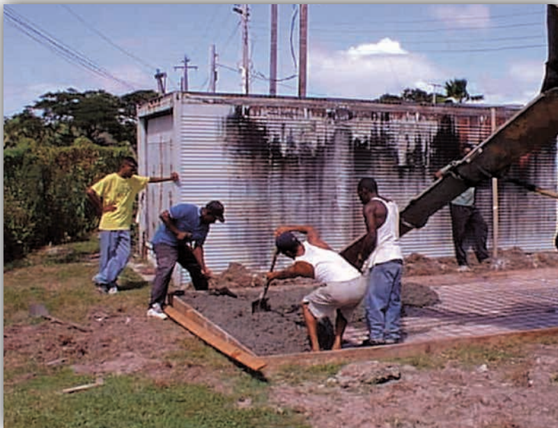
Pouring slab for storage unit at DMH
